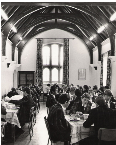
Hostel's elegant dining room . . . later part of matric exam headquarters, now a police complex
